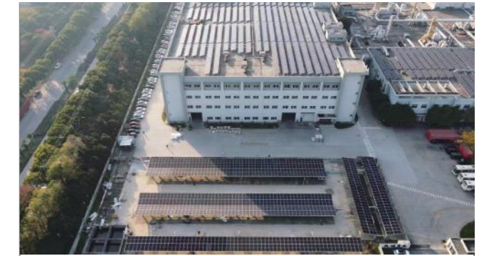
Jingpeng New Distributed PV Project 3.0MWp
