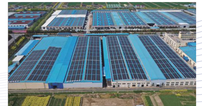
Fengguan Distributed PV Project 3.0MWp
