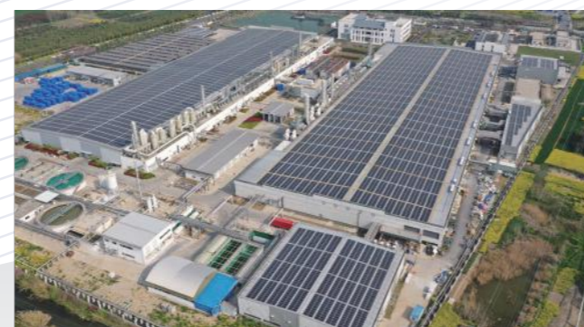
Runergy Yueda Distributed PV Project 7.4MWp
