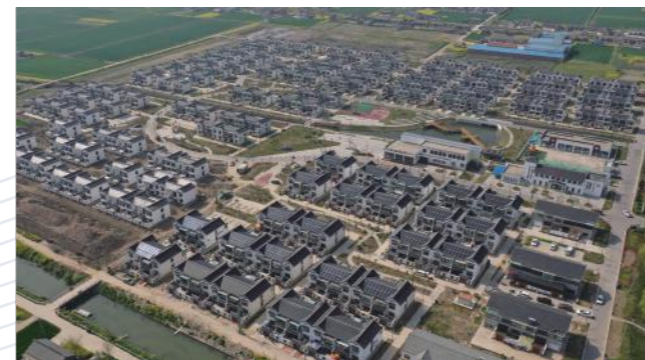
Bufeng Town Distributed PV Project 0.8MWp
