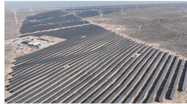
Pingluo Hongyazi PV Project 100MWp
