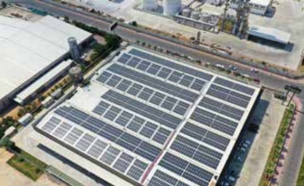
ANTALYA OSB 880 kWp - 2020
