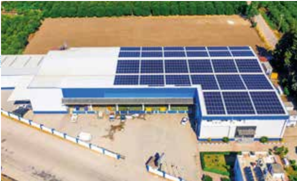
ANTALYA KUMLUCA 376 kWp - 2021
