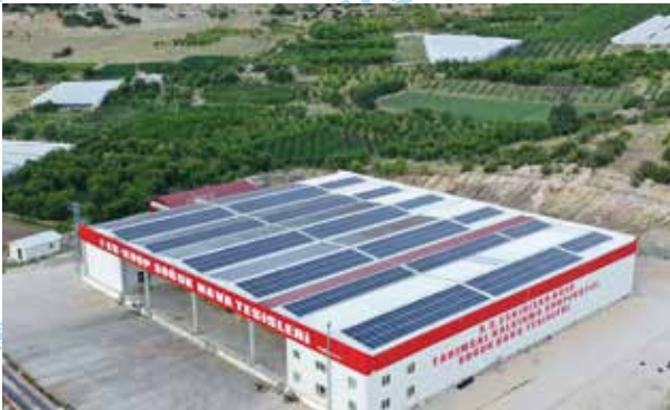
ANTALYA ELMALI 324 kWp - 2018
