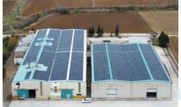
BALIKESİR BANDIRMA 720 kWp - 2021
