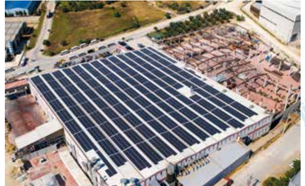
BURSA OSMANGAZİ 1.1 MWp - 2019
