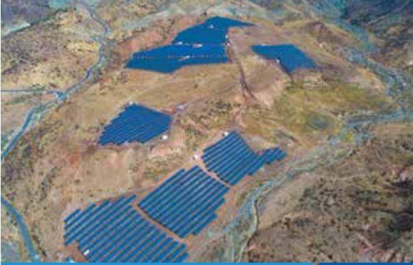
BATMAN KOZLUK 9.3 MWp - 2018
