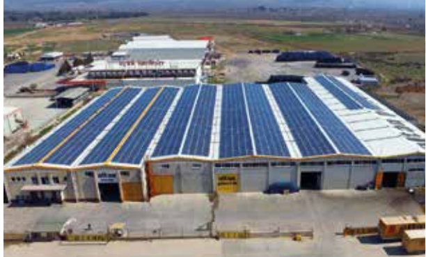
MANİSA ALAŞEHİR 1 MWp - 2016
